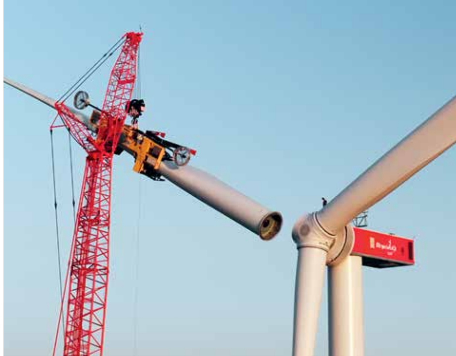
A new lifting device is used to install the rotor blades. This device uses two propellers to grip the rotor blades and automatically holds them in position during the installation process.
