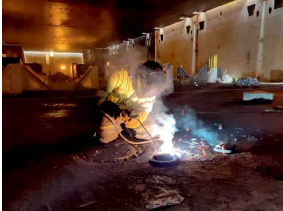
The lashing chains and metal plates used to secure the cargo are welded directly onto the ship and the cargo itself to prevent it from sliding around during the sea voyage.
