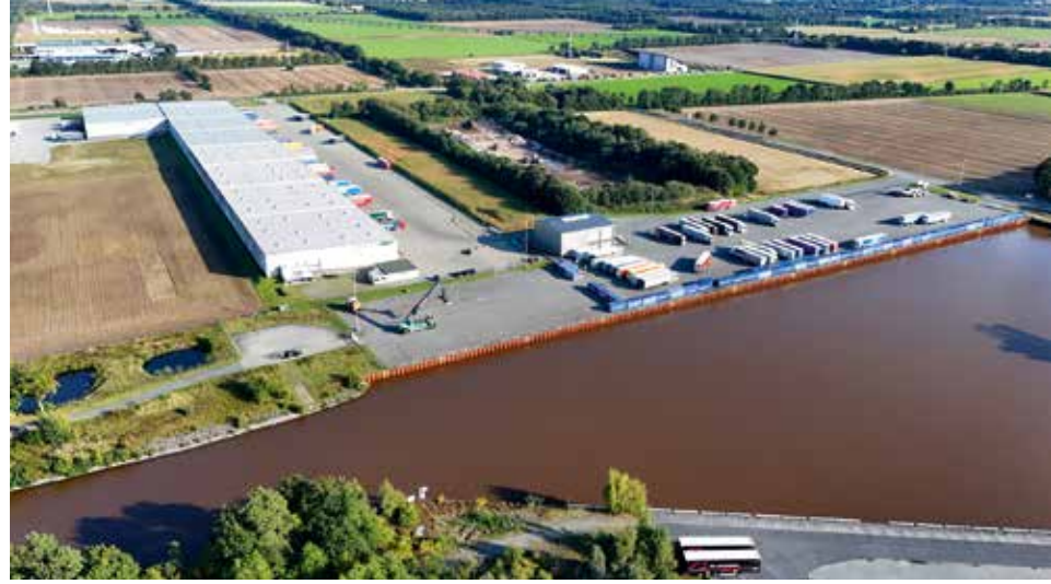
DUK has operated an intermodal transport facility with container transshipment and warehousing in Dörpen since 1989 and currently has 20,000 square metres of warehouse space.
