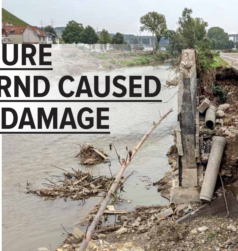
Flooded roads, collapsed houses and towns that were cut off: storm "Bernd" left a trail of destruction in parts of Germany.
